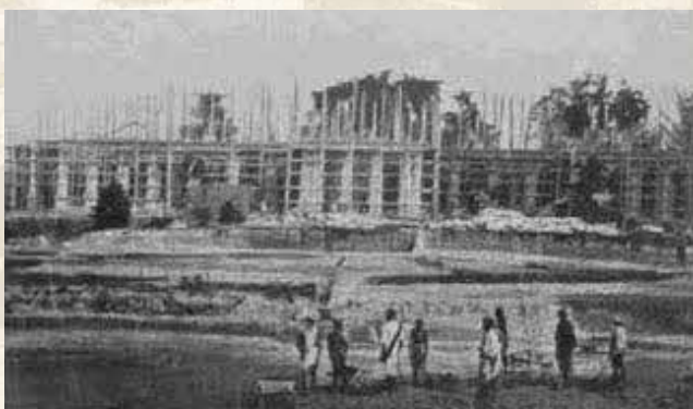
Government House garden being laid out by convicts
